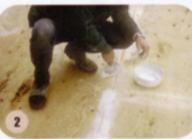
2 The surface must be smooth. This is accomplished by applying a special floor levelling compound mixed with latex to plywood joints, knot holes, uneven spots. On other surfaces such as concrete, surface must be ground smooth or levelled with a floor compound. Painted surfaces must be free of flaking paint. Note: Do not apply over treated plywood as chemicals may react with adhesives or PVC membrane.
