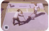
11 Seams are overlapped and heat welded together to provide a permanent bond. This method should be followed whenever two or more pieces of vinyl are required. The pieces should be overlapped by at least 3/4" and heat welded with a hot air welder. The PVC membrane is then heat welded to flashing and trimmed flush
