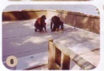
6 The PVC membrane is stapled in position, only on the seams. Later the staples will be removed and seams will be sealed using either a chemical sealer or hot air welding tool.
