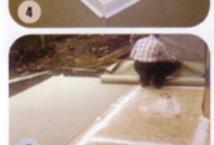
5 The vinyl is laid in place and stapled at the seams to prevent shifting during installation. The vinyl is overlapped the same direction as shingles on a roof. An allowance of 1" of vinyl is required going over the edge of the deck and 6 inches up the
