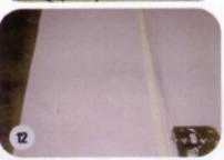
sealer: overlap seams by approx. 1 inch, mark off area with masking tape, and apply generous amount of chemical to lower piece of vinyl only. Immediately press both surfaces together. Place heavy object on top of seam such as 2 x 4 piece of wood and let stand overnight. Remove masking tape once seam is completed.
