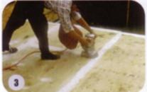
3 The deck is then sanded, usually with a disk sander or floor edger so that the area is as smooth as possible. Particular attention should be given to plywood joints.
